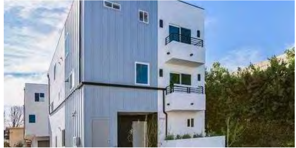
3 5261 Harmony Ave 5261 Harmony Ave North Hollywood, CA 91601
