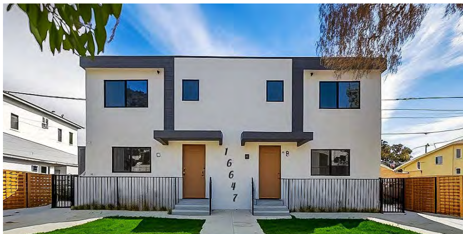
★ 16647 Victory Blvd 16647 Victory Blvd, Van Nuys, CA 91406
